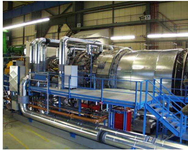
Figure 5: Siemens' W501FD Test Facility in Berlin, Germany (Wolfe and Antos 4)
